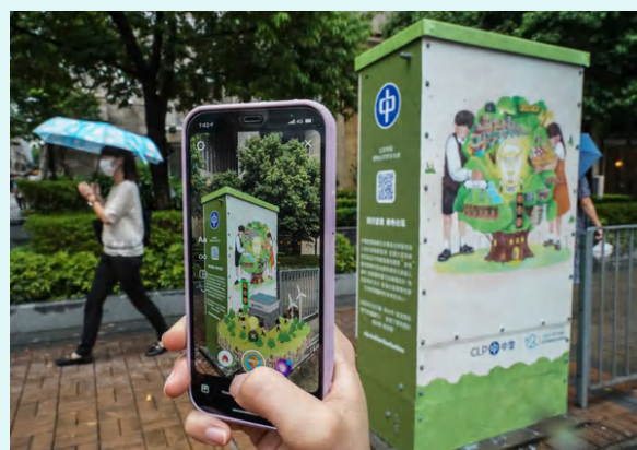
The distribution boxes also feature the ability to add sustainability-inspired effects to photos using augmented reality.
