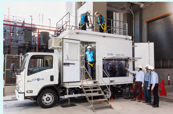
The Mobile Safety Training Workshop allows demonstration of confined space safety procedures in a controlled environment.
