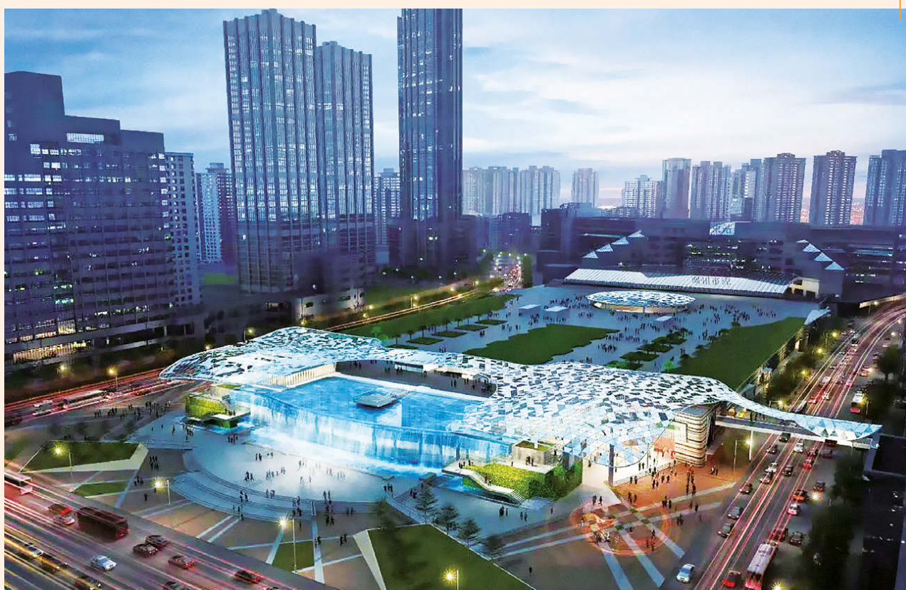
CLP began a comprehensive upgrade of the centralised cooling system at Po Park Shopping Plaza in Guangzhou in 2021 and will operate the retail complex's cooling services until 2036.
