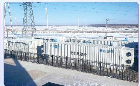
The 5MW battery energy storage system at Qian'an III Wind Farm
